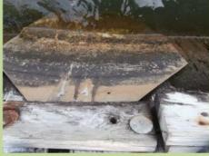
An example of what not to do: previously ordered work used stop sign to secure bulk head
